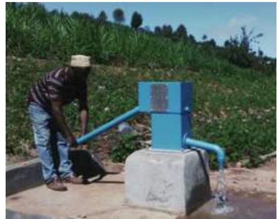
Inspections of the water pumps
