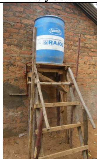
Water tank outside
