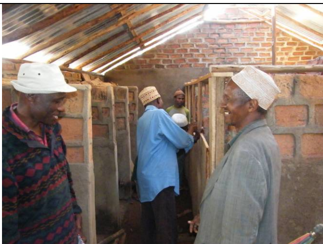
Inspection of the new girls toilet
